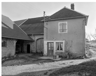
Partie habitation. Phot. Yves Sancey IVR43_19847000040X
