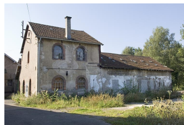
Atelier ouest. Phot. Jérôme Mongreville IVR43_20097000864NUC2A
