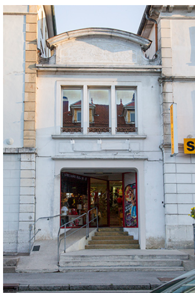
Porche. Phot. Yves Sancey IVR43_20132502374NUC2A
