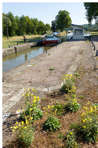
L'écluse. Phot. Sonia Dourlot IVR43_20157000729NUC2A
