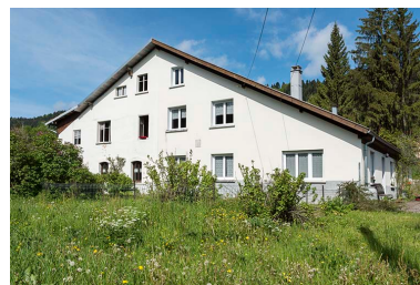
Elévation sud-est. Phot. Sonia Dourlot IVR43_20172500734NUC4A
