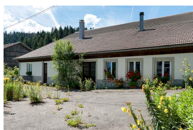
Elévation nord-est. Phot. Sonia Dourlot IVR43_20172500735NUC4A
