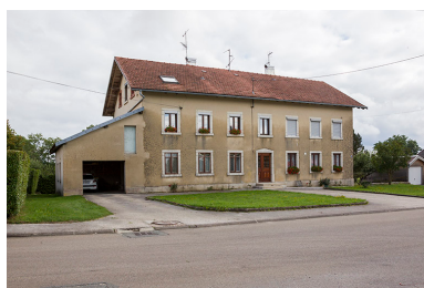
Façade antérieure. Phot. Yves Sancey IVR43_20132501347NUC2A
