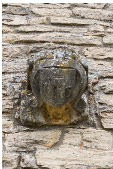
Phot. Pierre-Marie Barbe-Richaud IVR26_20237100229NUC4A
