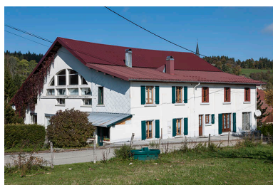
Scierie communale, Remoray-Boujeons. Phot. Jérôme Mongreville IVR43_20152501901NUC4A
