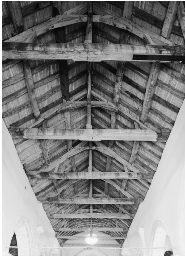
Charpente de la nef. Phot. Michel Thierry IVR26_19802100493V
