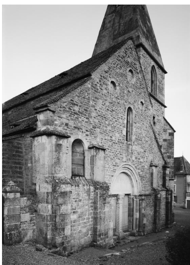
Façade. Phot. Michel Rosso IVR26_19782101426V
