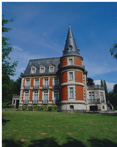
Façade ouest. Phot. Yves Sancey IVR43_20029000410XA
