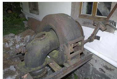
Turbine horizontale. Phot. Jérôme Mongreville IVR43_20057000266NUCA
