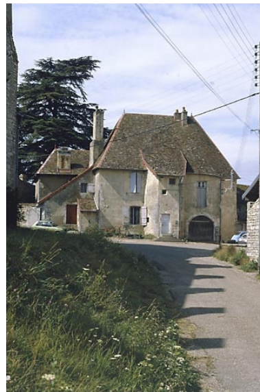
Façade antérieure Phot. Yves Sancey IVR43_19857000161XA
