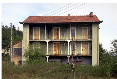
Logement. Phot. Laurent Poupard IVR43_19913901281ZA
