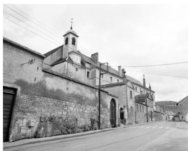
Elévation rue Edouard Bastide. Phot. Yves Sancey IVR43_19762501291X
