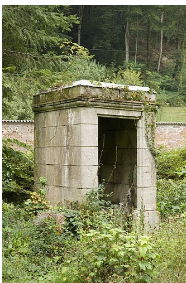
Latrines. Phot. Jérôme Mongreville IVR43_20067000701NUCA
