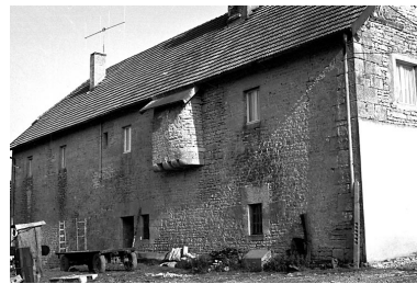
Façade postérieure. Phot. Gilbert Poinot IVR43_19752501396Z
