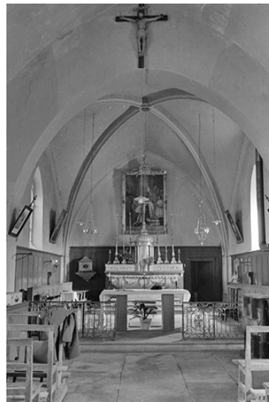
Choeur vu de la nef. Phot. Guy Forestier IVR43_19743900444Z
