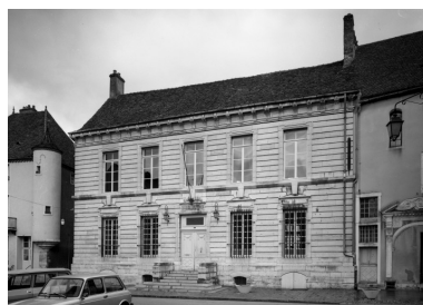
Façade. Phot. Michel Rosso IVR26_19862100093V
