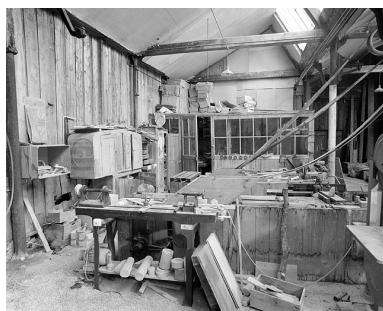
Atelier de menuiserie. Phot. Yves Sancey IVR43_20022500736X
