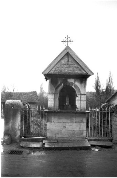
Vue de face. Phot. Guy Forestier IVR43_19743900365Z
