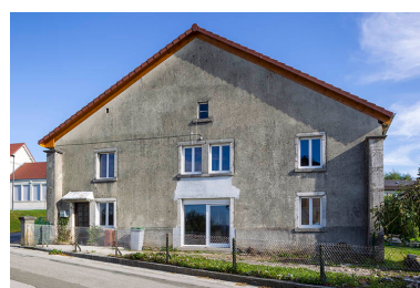
Façade antérieure. Phot. Sonia Dourlot IVR43_20152500923NUC2A
