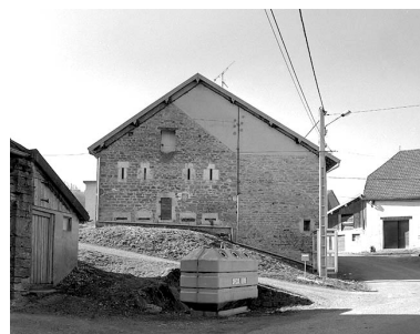
Façade nord. Phot. Yves Sancey IVR43_19973900557X
