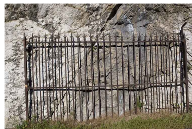
Grille vue de face. Phot. Yves Sancey IVR43_20062500151NUCA
