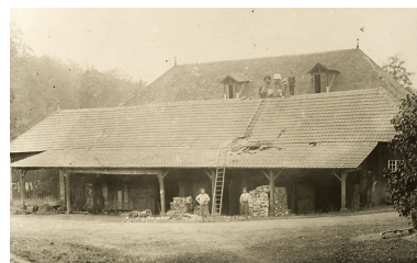
Atelier de forge (?). Phot. Jérôme Mongreville IVR43_20077000079NUCA
