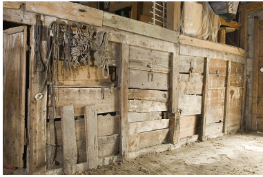
Grange. Phot. Jérôme Mongreville IVR43_20082500795NUC2A
