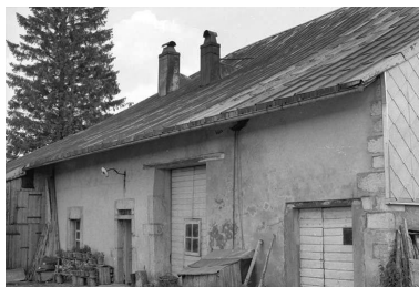
Façade postérieure. Phot. Gilbert Poinot IVR43_19752500988Z
