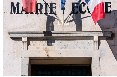
Inscription surmontant la porte principale. Phot. Jérôme Mongreville IVR43_20152502377NUC4A
