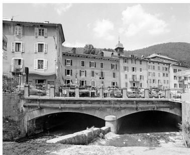
Tête amont. Phot. Yves Sancey IVR43_20033900625X
