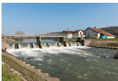
Barrage mobile, Cendrecourt. Phot. Sonia Dourlot IVR43_20167000263NUC4A
