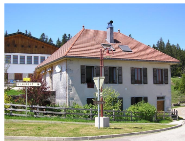
Ecole. Phot. Marie-Pierre Reynet IVR43_20083900293NUC1A
