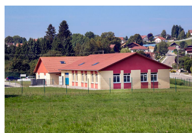
Atelier est. Phot. Yves Sancey IVR43_20132501386NUC2A
