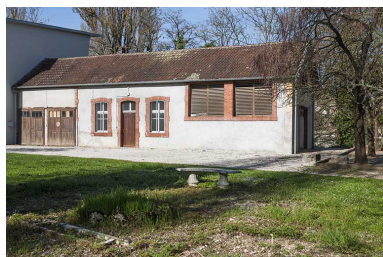
Annexe (buanderie, séchoir). Phot. Jérôme Mongreville IVR43_20132500146NUC4A
