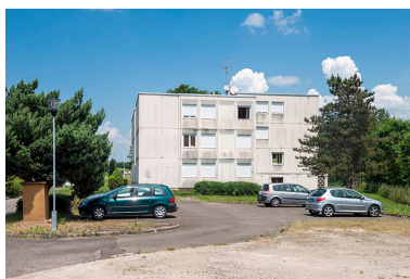
Façade sud des logements. Phot. Mary Ruffinoni IVR43_20147000111NUC4A
