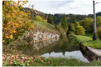
Bassin de retenue. Phot. Sonia Dourlot IVR43_20172501780NUC4A
