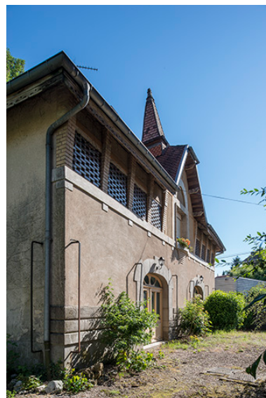
Façade principale. Phot. Jérôme Mongreville IVR43_20187000471NUC4A
