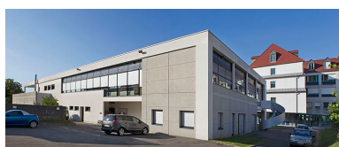
Restauration : façade Est. Phot. Sonia Dourlot IVR43_20143900746NUC2A
