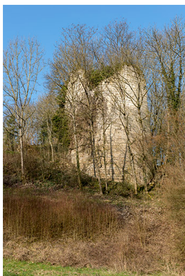
Tour nord en ruine. Phot. Sonia Dourlot IVR43_20167000659NUC4A
