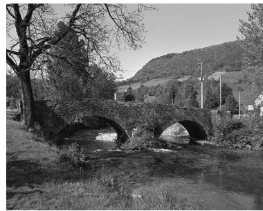
Face amont. Phot. Yves Sancey IVR43_19813900219X
