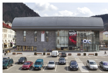
Façade antérieure. Phot. Yves Sancey IVR43_20103900163NUC2A
