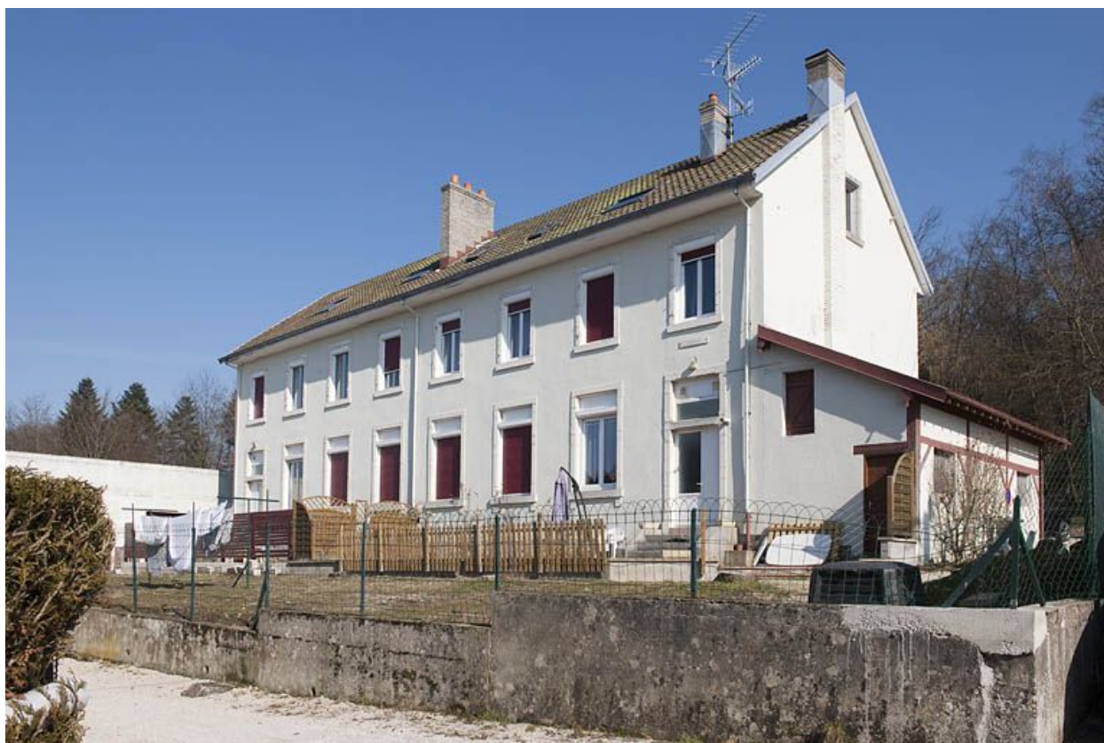
Ecole. Façade ouest.
