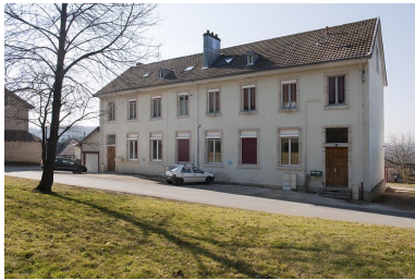
Ecole. Façade est. Phot. Jérôme Mongreville IVR43_20122500151NUC4A
