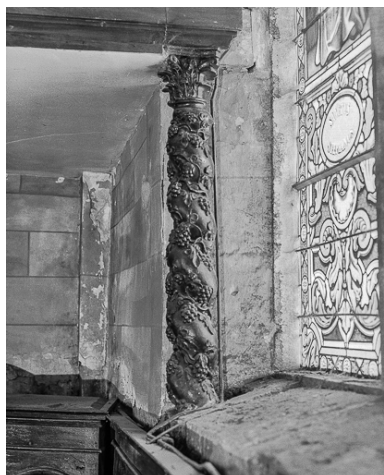
Colonne torsée soutenant la tribune. Phot. Yves Sancey IVR43_19742500705X
