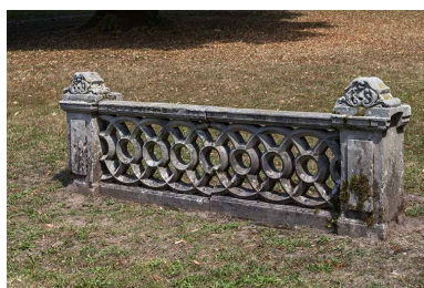
Garde-corps. Phot. Jérôme Mongreville IVR43_20207000401NUC4A
