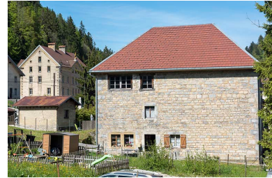
Façade occidentale. Phot. Sonia Dourlot IVR43_20172500442NUC4A
