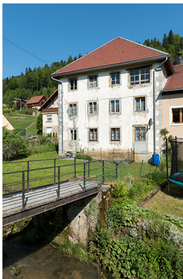
Façade sud. Phot. Sonia Dourlot IVR43_20172500441NUC4A
