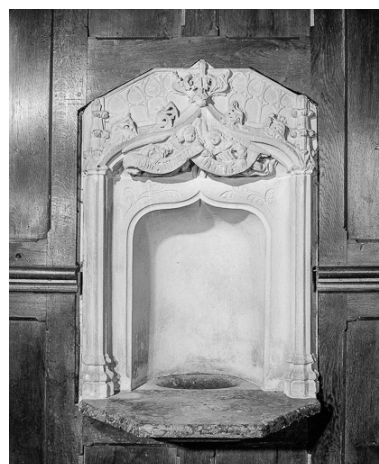
Niche. Phot. Yves Sancey IVR43_19767000682X
