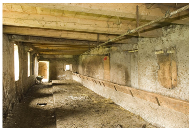
Etable. Phot. Jérôme Mongreville IVR43_20082500963NUC2A
