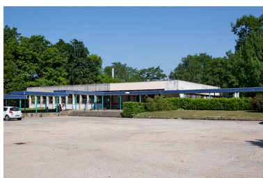
Façade sud de la cantine. Phot. Sonia Dourlot IVR43_20142500941NUC2A
