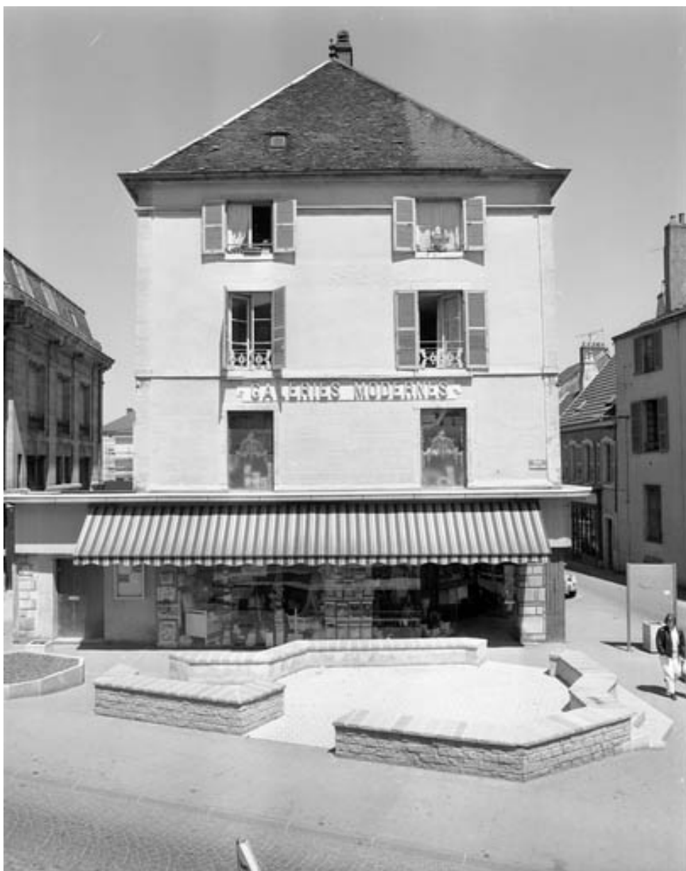
Façade principale, de face.
