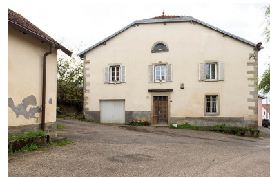
Vue de face : pignon est. Phot. Sonia Dourlot IVR43_20157001374NUC4A
