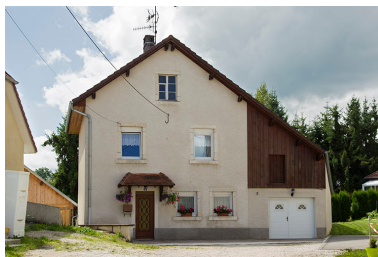
Façade antérieure. Phot. Sonia Dourlot IVR43_20142501802NUC2A
