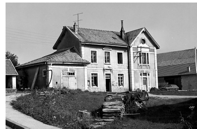
La fromagerie Phot. Yves Sancey IVR43_19802500864V
